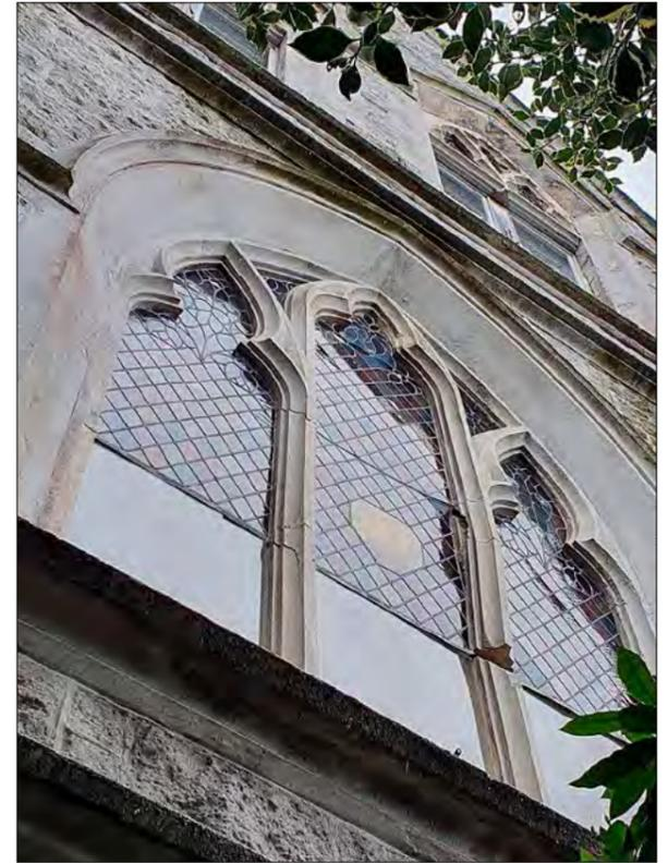
The window in place, with one of the mullions broken and cracked, and no longer supporting the weight bearing down from above.
